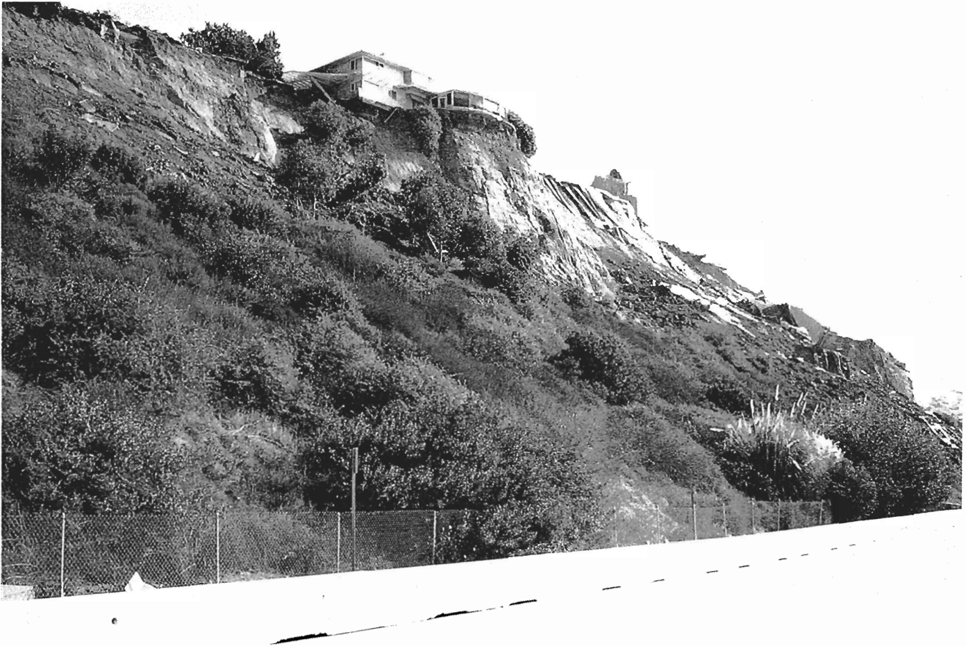
Above: Landslides along the Pacific Coast Highway, between Santa Monica and Pacific Palisades
